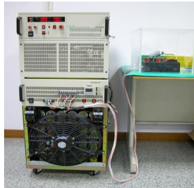
Fault Current Test
